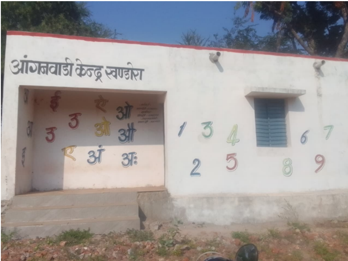
The Anganwadi Centre of Khandora village after the completion of construction work. (Photo Credit: Dhuleshwar Pargi, Community Facilitator, Vaagdhara)
