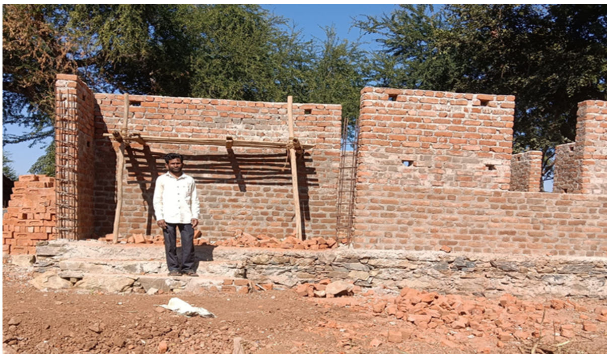
The Anganwadi Centre of Khandora village after the completion of construction work. (Photo Credit: Dhuleshwar Pargi, Community Facilitator, Vaagdhara)
