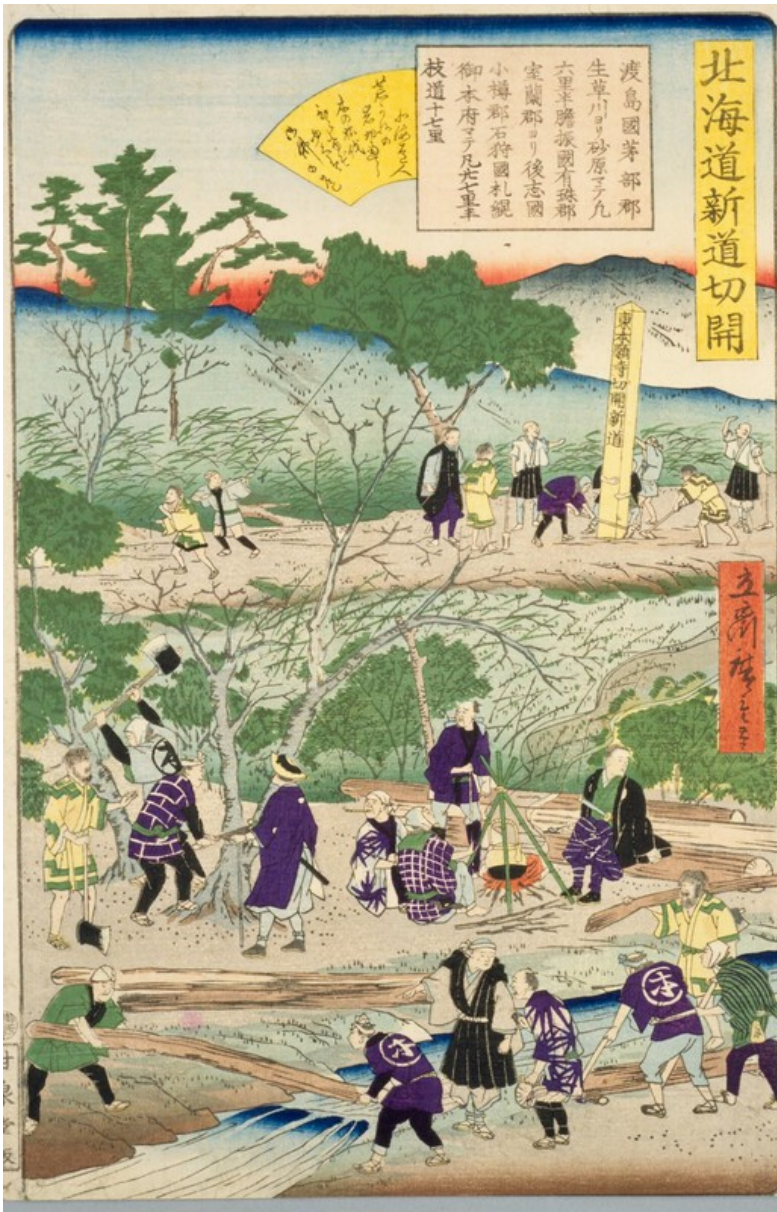
Figure 2: The opening of a new highway in Hokkaidō through the temple named Higashi Honganji. Ainu workers are depicted wearing beards and yellow clothes decorated with geometrical patterns. Source: Hokkaidō shindō sekkai (北海道新道切開) 1871 © National Diet Library.
