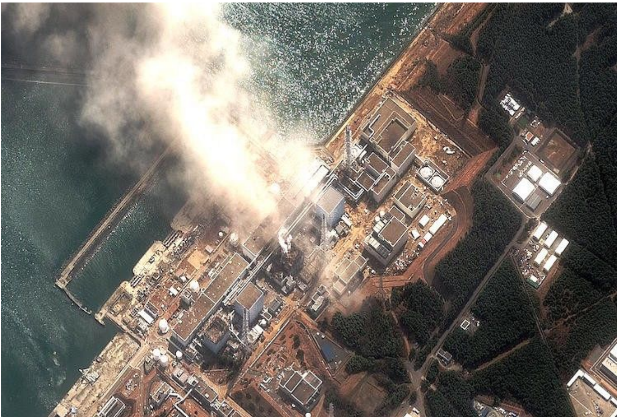
Satellite image shows damage at Fukushima Nuclear Power Plant (via ecowatch.com).
