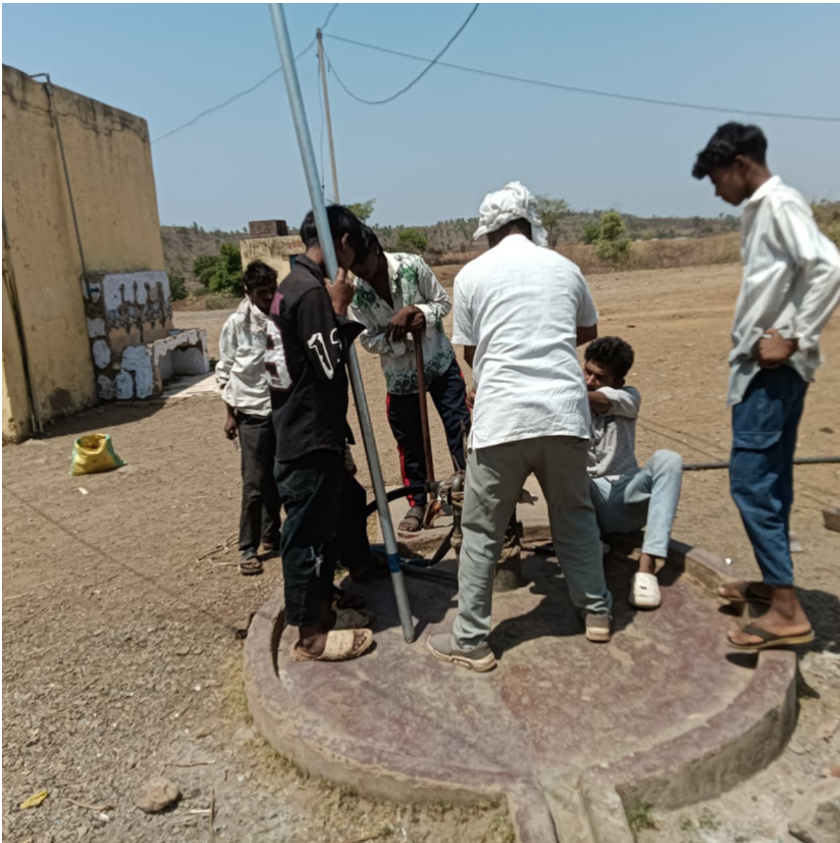
Repair work under way in one of the 18 villages covered by the Sangathan's survey. (Photo: Mohan Bhuria, Sangathan Coordinator, VAAGDHARA)
