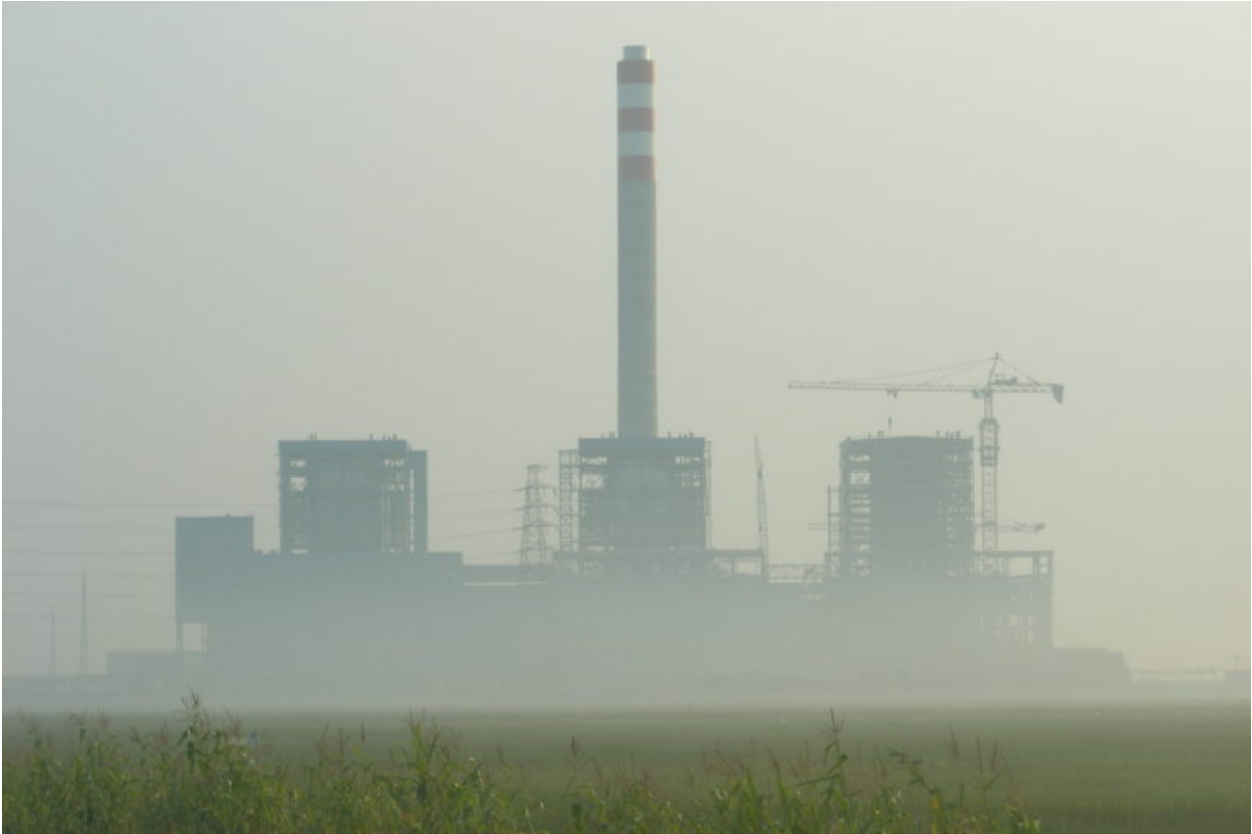
Coal-fired power plant in Indramayu, West Java, Indonesia. Image by Bkusmono/Wikimedia Commons.
