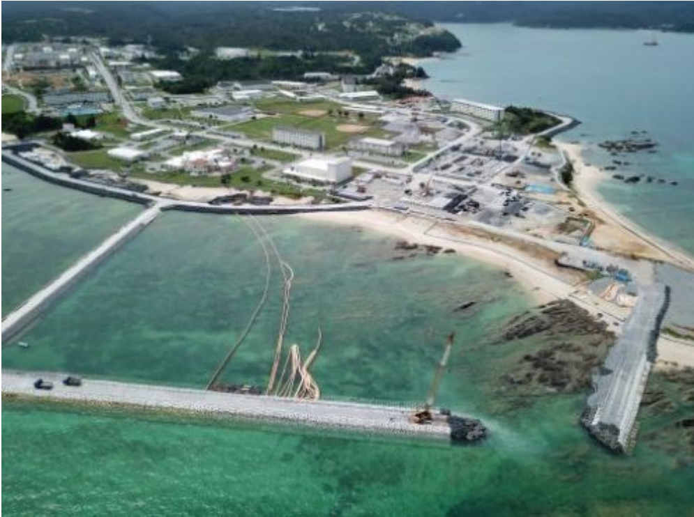
Sea Wall Construction at Henoko, Ryukyu shimpo, 19 July 2018.
