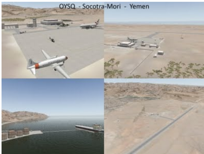
Existing runway and airport
